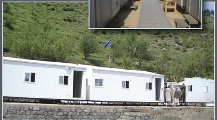
Photo: D&D - FRB (Fast Response Building)
